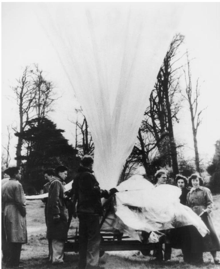
**Figure 1** A balloon ready for the ascent in the Sardinia area in July 1953. For the first time, emulsion stacks were made up of 40 stripped emulsions bound together between thick glass plates, wrapped and sealed and subsequently marked with X-rays.
